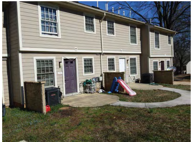
Typical Subject building
