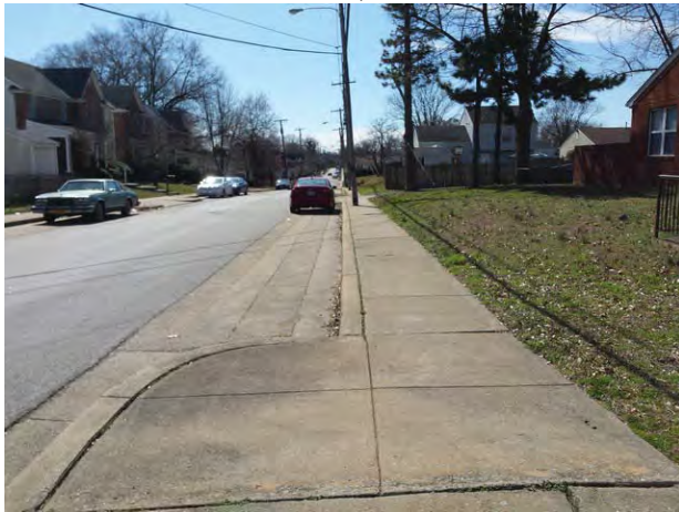
View along Allen Avenue looking south (Subject to the right)
