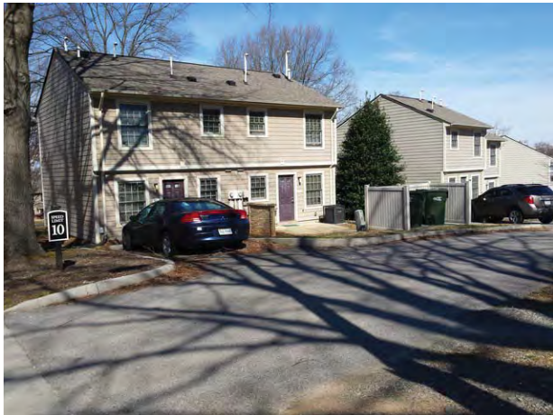
Typical Subject buildings from interior of site
