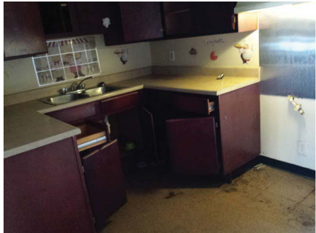
Typical kitchen - vacant unit
