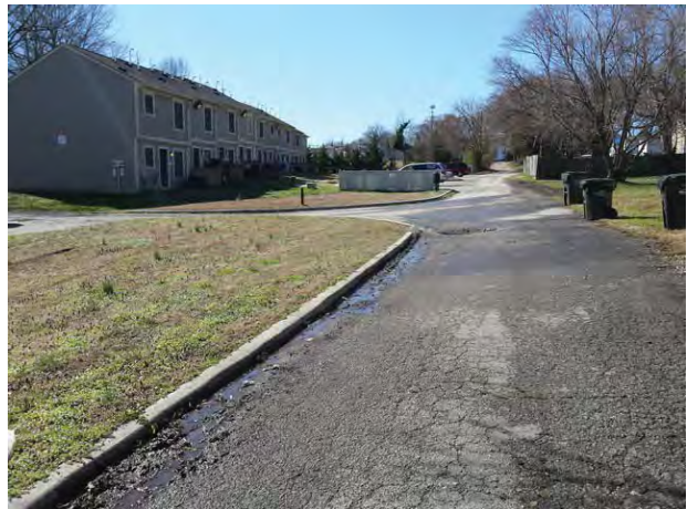
Interior access road to the rear of Subject site
