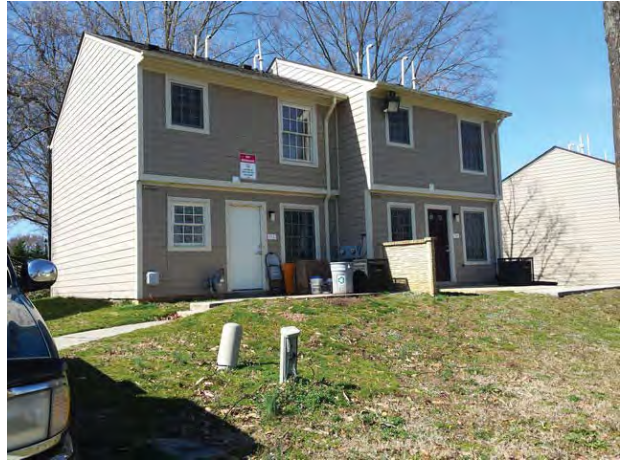
Typical Subject building from interior of site
