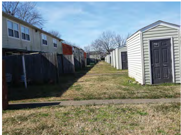
Rear yard and storage sheds of typical Subject building
