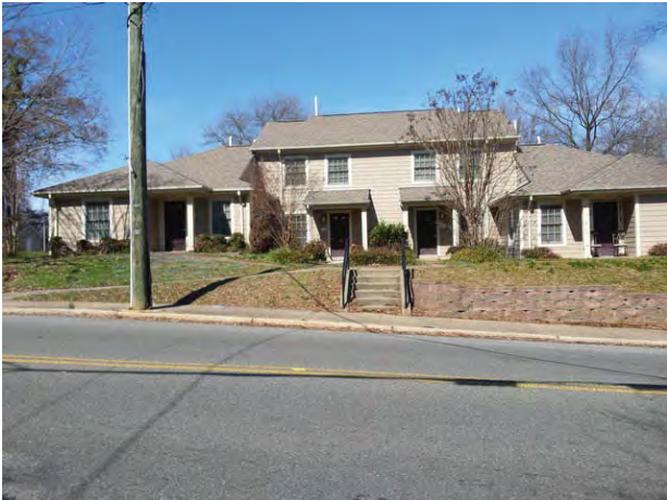
Subject from Bainbridge Street looking north
