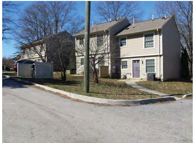
Typical Subject building from interior of site
