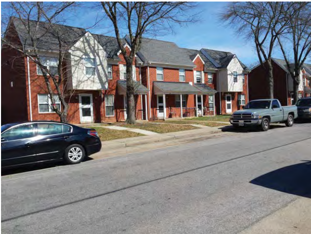
Typical Subject building from Idlewood Avenue looking northeast
