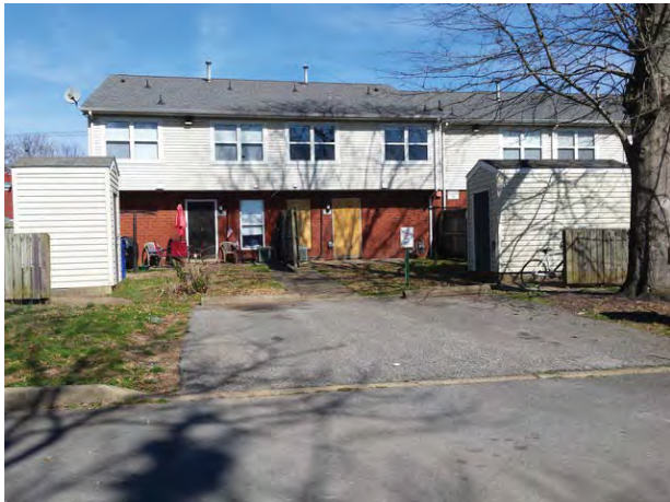
Rear of typical Subject building
