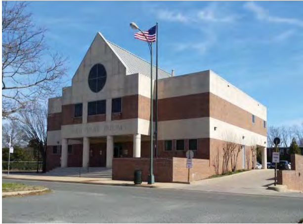
Police station along South Meadow Street to the north of Subject
