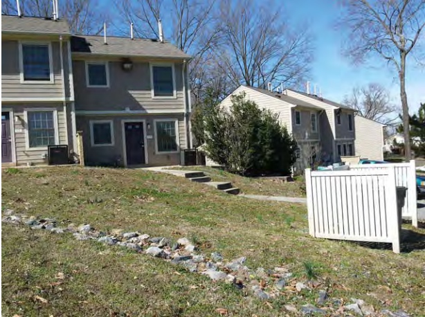
Typical Subject building from interior of site
