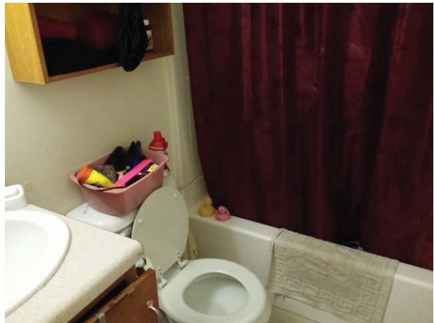
Typical bathroom – occupied unit
