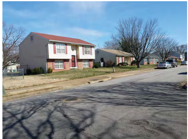
Single-family homes along Rosewood Avenue to the south of Subject
