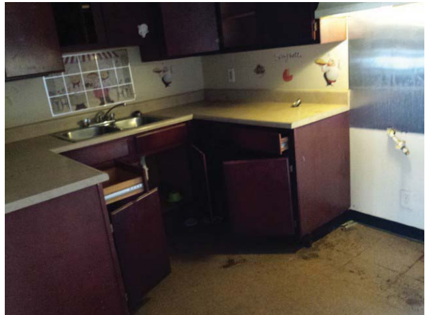
Typical kitchen – vacant unit
