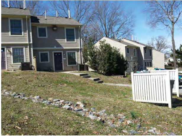
Typical Subject building from interior of site
