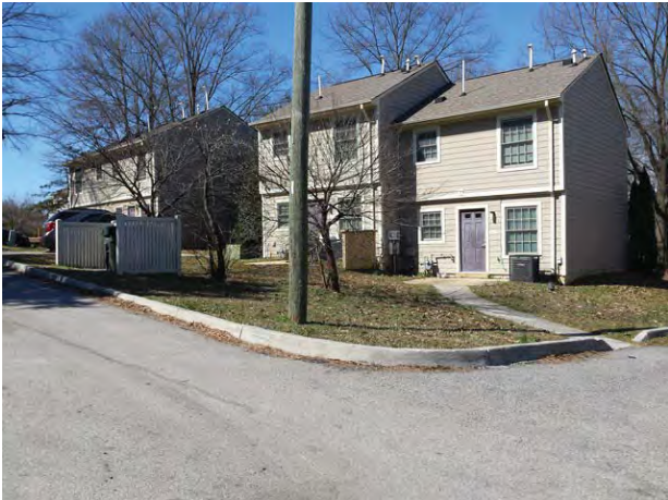
Typical Subject building from interior of site
