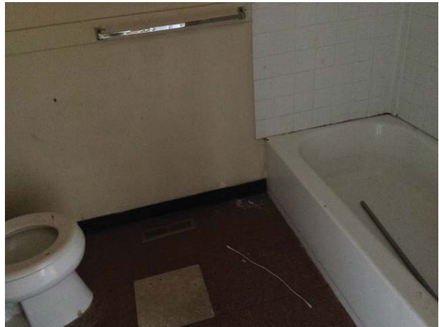
Typical bathroom – vacant unit
