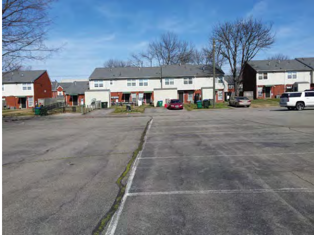
Subject from parking area of house of worship looking north
