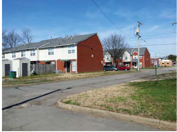
Typical Subject buildings looking north from adjacent ally
