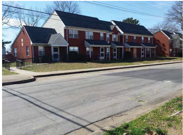
Typical Subject building from Idlewood Avenue looking southwest
