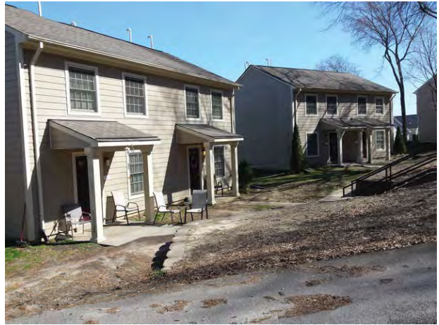
Typical Subject building from interior of site
