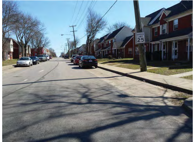
View along Idlewood Avenue looking east (Subject on both sides of street)
