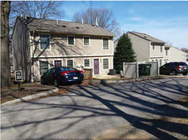
Typical Subject buildings from interior of site
