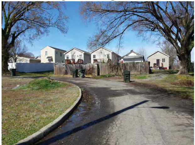
Rear of adjacent single-family homes along Perry Street to the north of Subject
