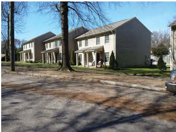
Typical Subject building from interior of site
