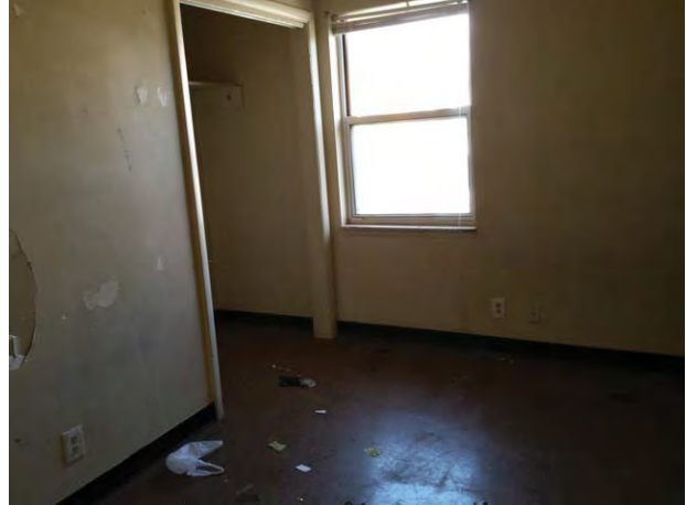
Typical bedroom – vacant unit
