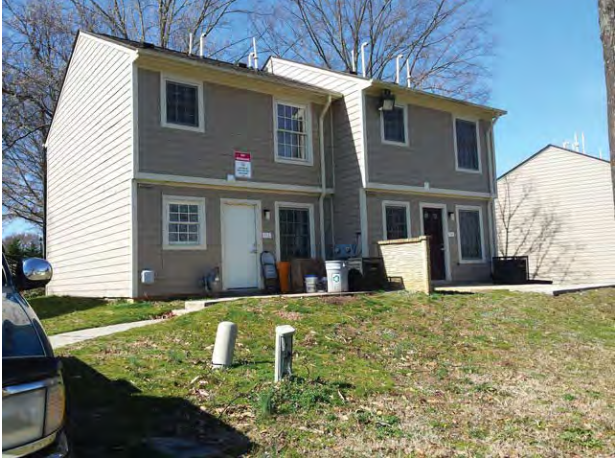
Typical Subject building from interior of site
