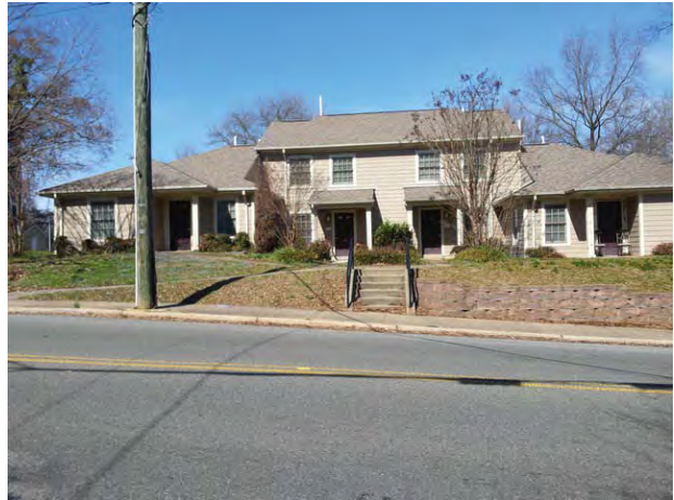
Subject from Bainbridge Street looking north
