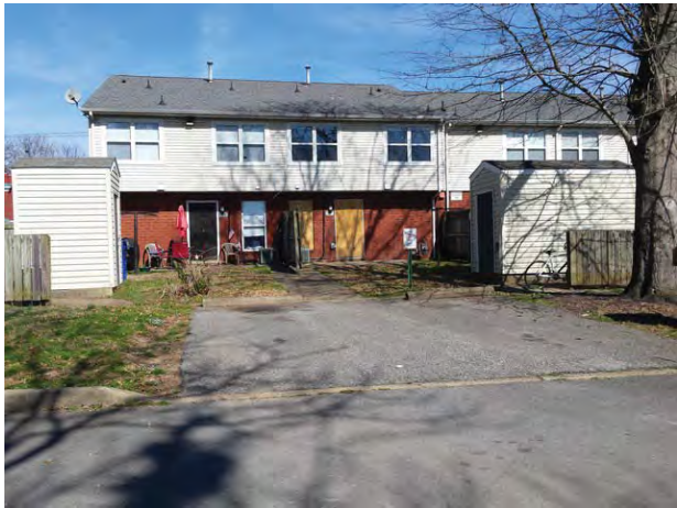
Rear of typical Subject building
