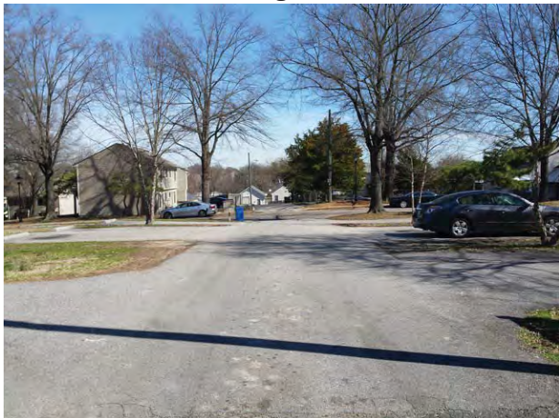
Interior access road and parking area
