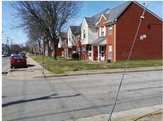
Typical Subject building from Idlewood Avenue looking west
