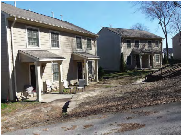
Typical Subject building from interior of site
