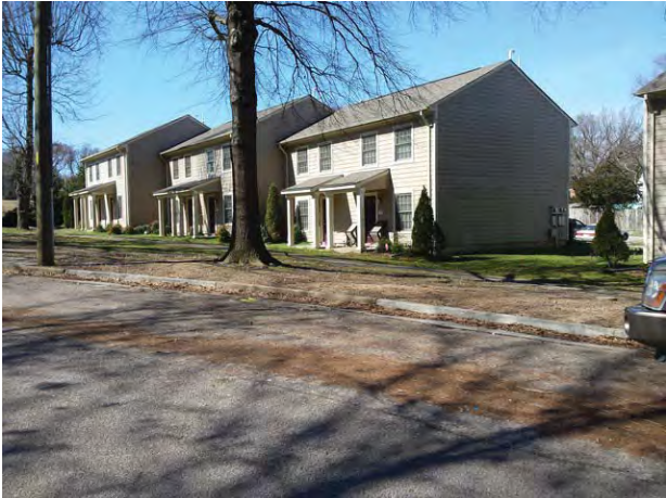
Typical Subject building from interior of site
