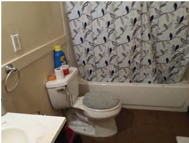
Typical bathroom – occupied unit
