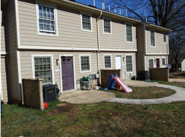
Typical Subject building
