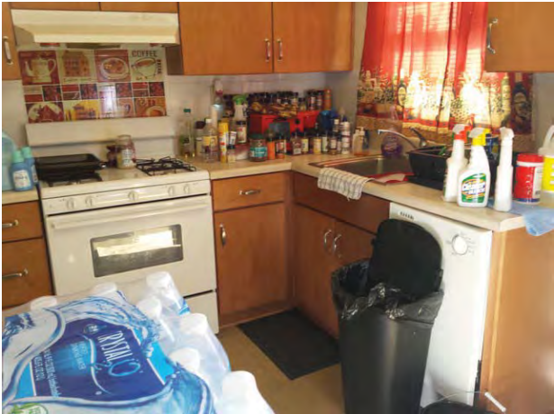
Typical kitchen – occupied unit
