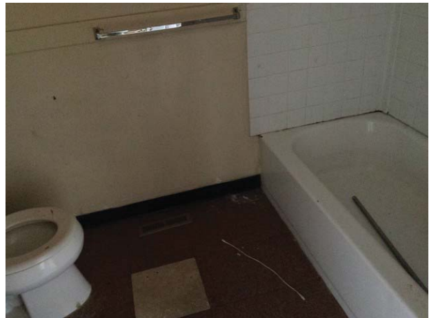
Typical bathroom – vacant unit
