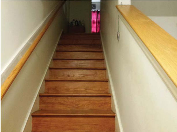
Typical interior stairway – occupied unit
