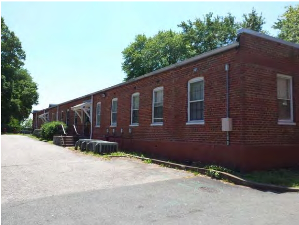
Rear of Subject Shockoe III building
