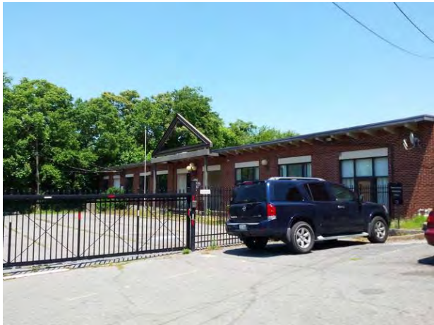
Adjacent vacant commercial building slated to be Subject community space
