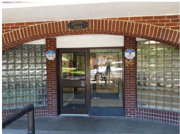
Alternative view of Shockoe I building entrance area
