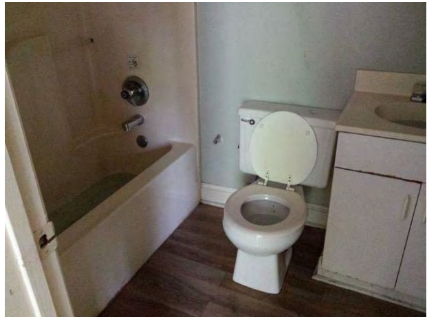
Typical bathroom – vacant unit
