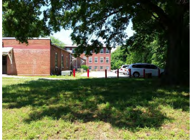
Parking area behind Shockoe III building
