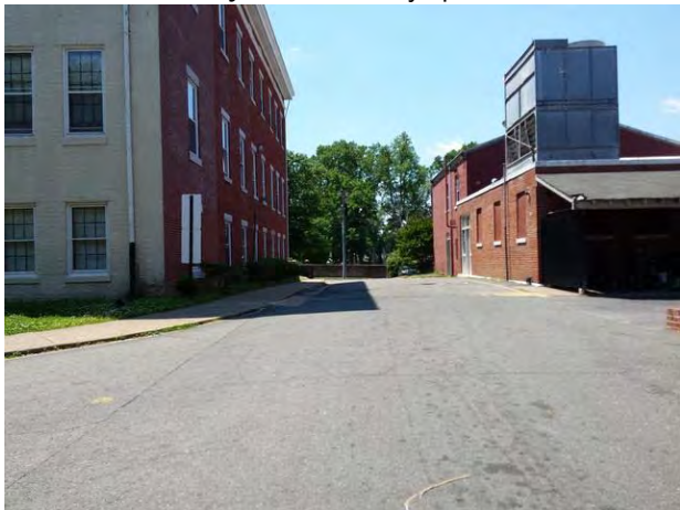
Subject entryway looking south (Shockoe I building to the left, utility building to the right)
