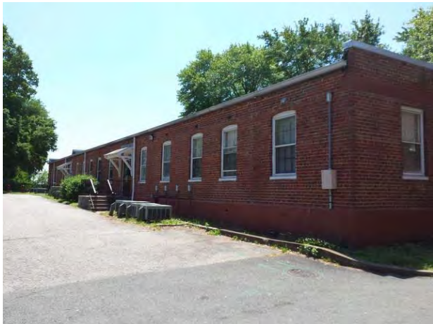
Rear of Subject Shockoe III building
