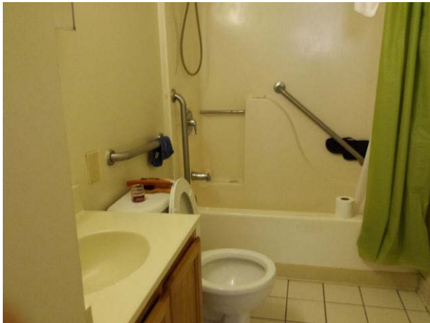
Typical bathroom – occupied unit
