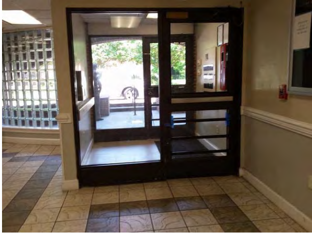
Interior entrance area
