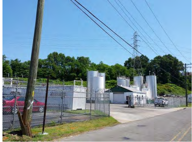
Industrial uses to the north of Subject along Valley Road
