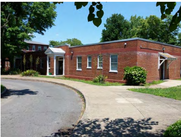
Alternative of View of Subject Shockoe III building
