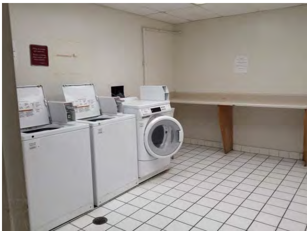
Central laundry room
