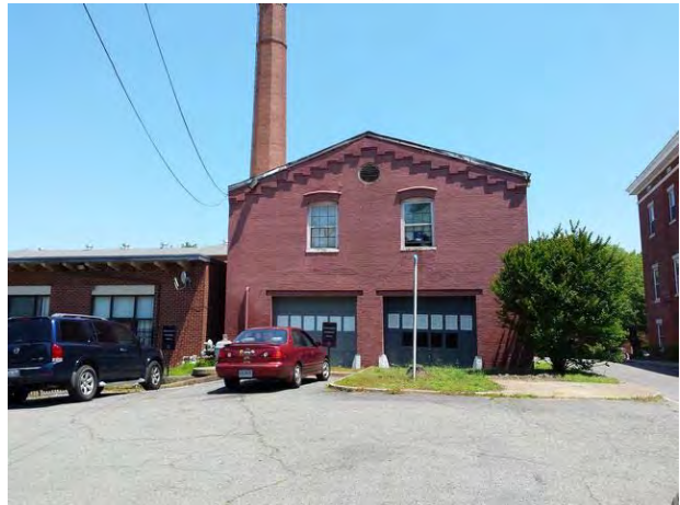
Alternative view of vacant commercial building on the left and utility building on the right
