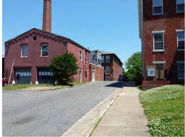
Entrance with Subject Shockoe I building on the right and utility building on the left
