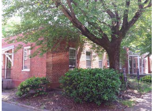
View of Subject Shockoe III building
