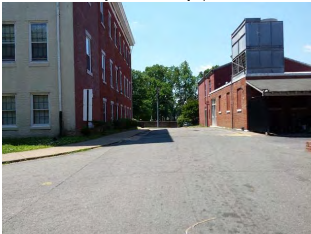
Subject entryway looking south (Shockoe I building to the left, utility building to the right)
