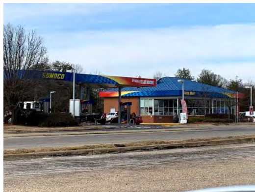
Further south of site, Sunoco gas station on Annapolis Way.
