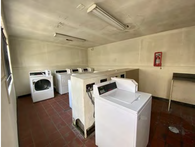
Subject laundry room (will be demolished)
