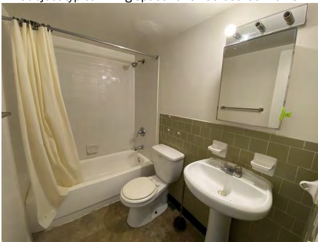
Subject typical bathroom for three-bedroom unit
