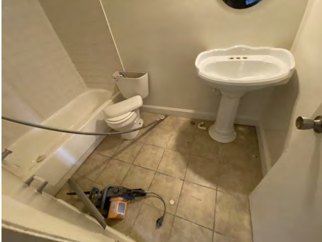
Subject typical bathroom for one-bedroom unit
