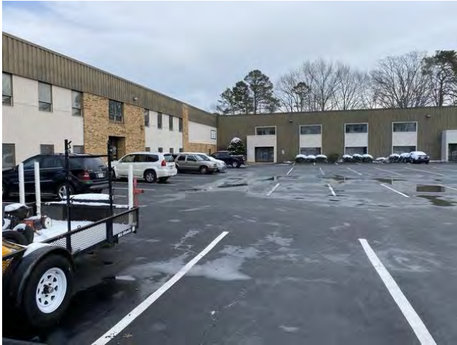
Office building south of the Subject
