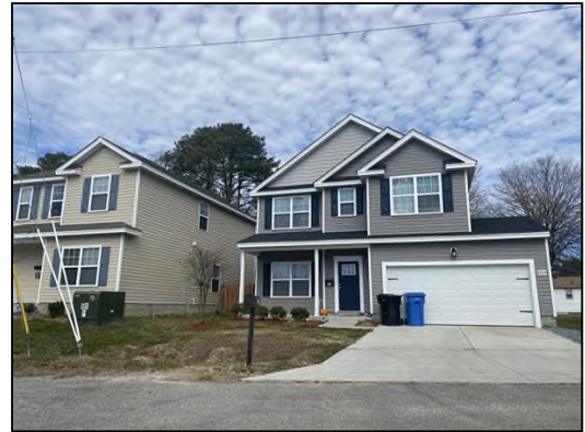
Single family homes north of subject site
