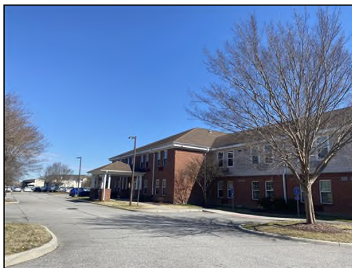
Offices across from subject site
