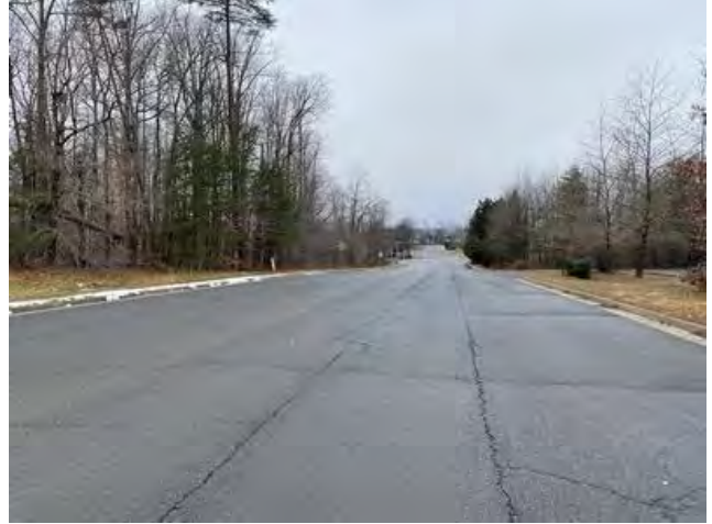
View west along Autumn Willow Drive
