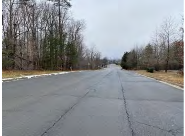
View west along Autumn Willow Drive
