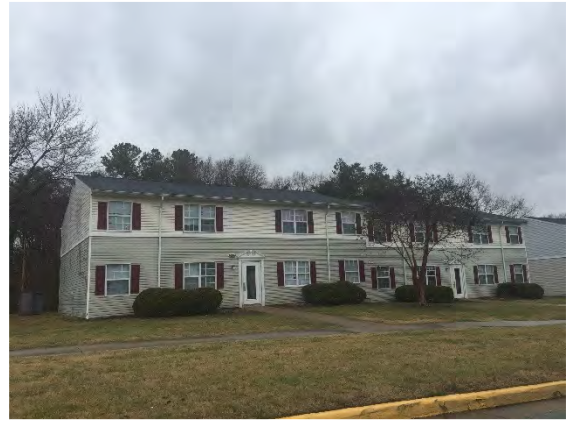
South Pointe Landing
