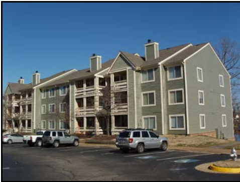
Waterside at Ironbridge
