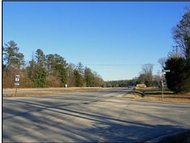
View east on Iron Bridge Rd., at W. Booker Blvd.
