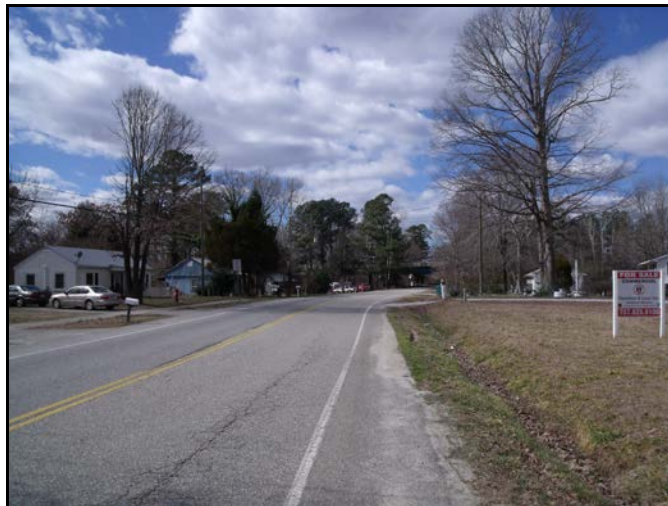
View west on Old Mooretown Rd., at site
