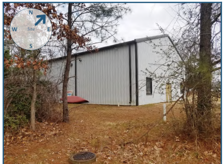
Northeast view from site
