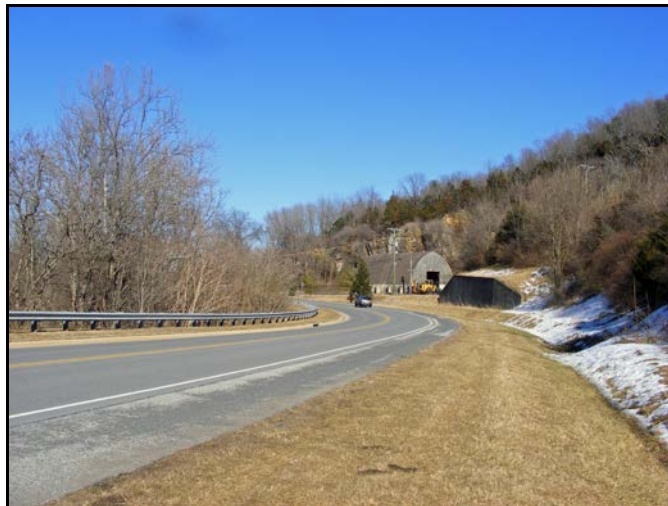
View north on Middlebrook Ave., at site
