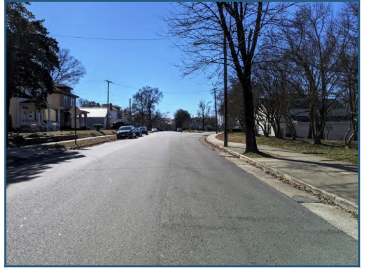
Streetscape: South view of 2nd Avenue
