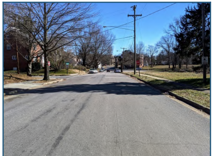
Streetscape: East view of Fourquare Lane
