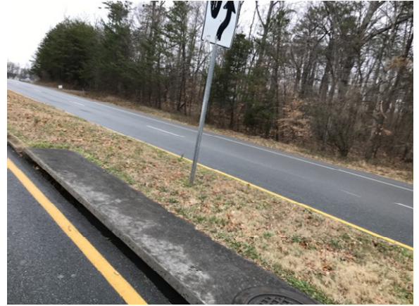
Looking northeast at site from Old Lynchburg Road
