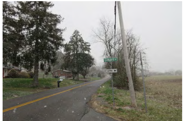
Looking South From Entrance
