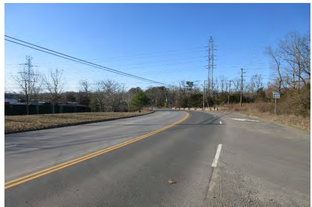
Looking West From Entrance
