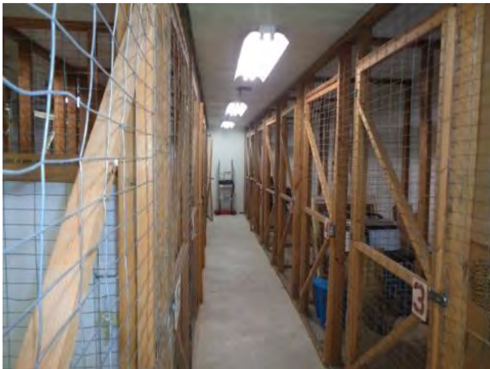
View of Exterior Storage
