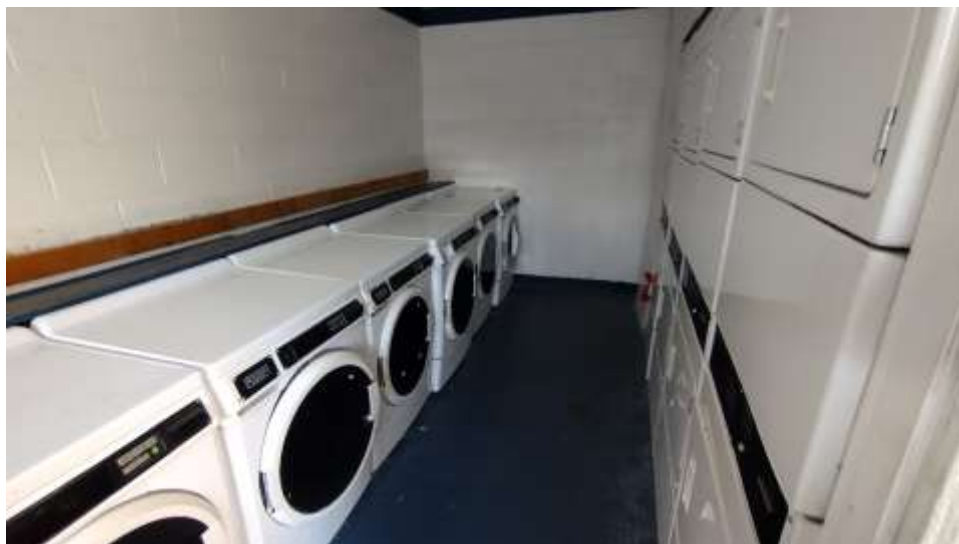
View of Laundry Facility
