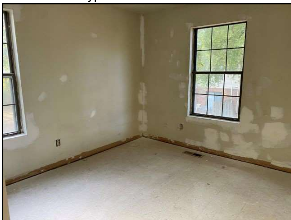
View of typical bedroom in vacant unit
