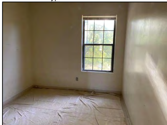
View of typical bedroom in vacant unit
