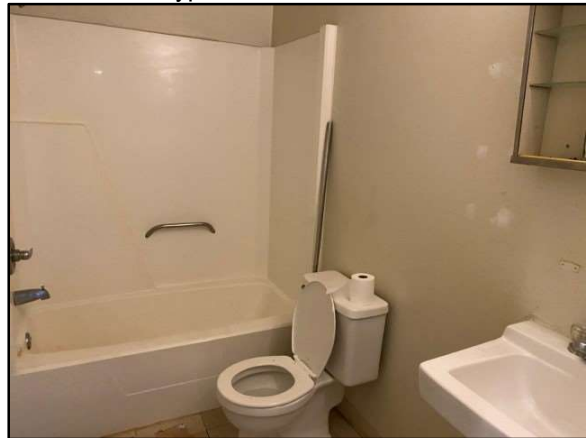
View of typical bathroom in vacant unit
