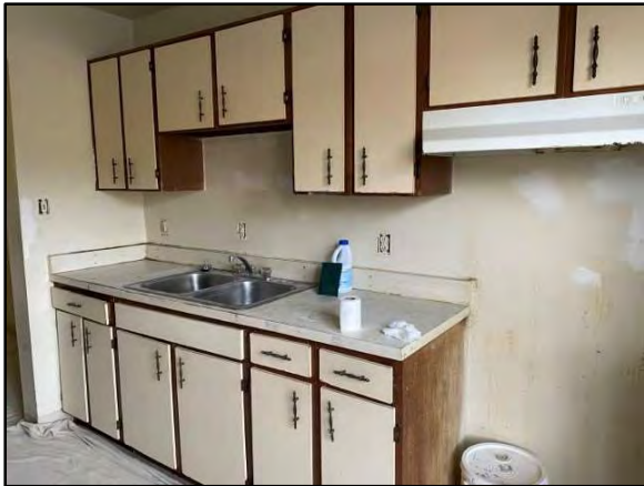
View of typical kitchen in vacant unit
