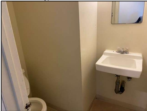
View of typical bathroom in vacant unit
