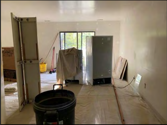
View of typical living room in vacant unit
