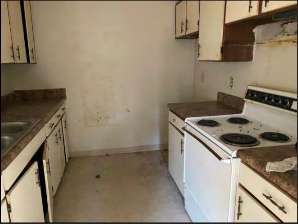
View of typical kitchen in vacant unit
