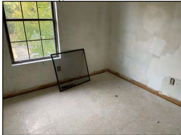
View of typical bedroom in vacant unit
