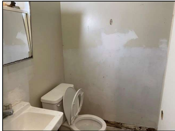
View of typical bathroom in vacant unit
