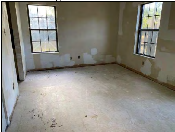
View of typical bedroom in vacant unit
