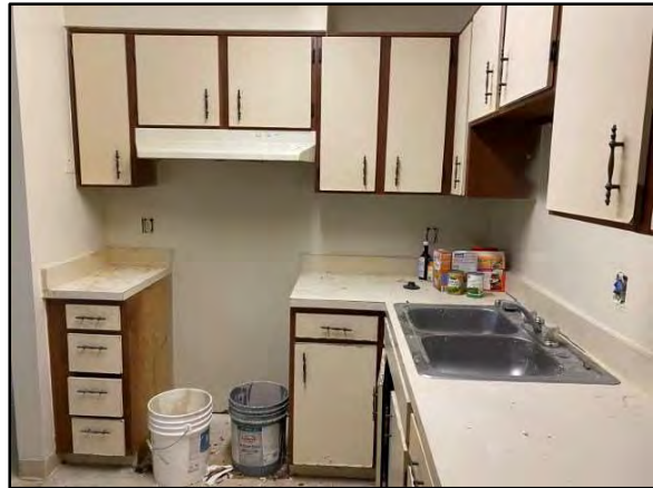
View of typical kitchen in vacant unit
