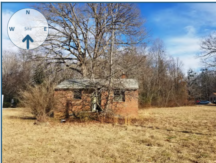
View of site from the south
