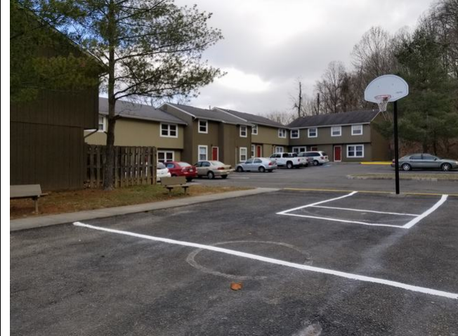
SUBJECT BASKETBALL COURT AND EXTERIOR
