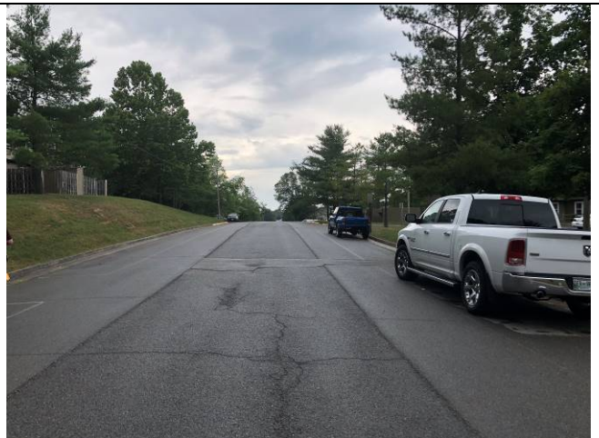
VIEW NORTH ON FAIRFAX STREET
