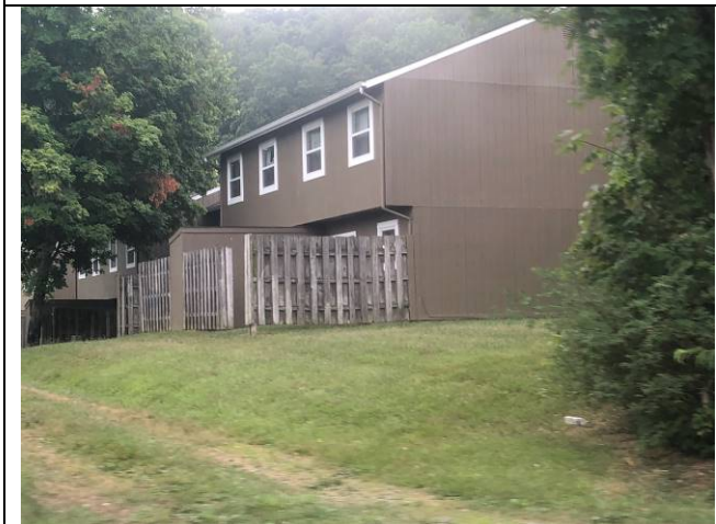
SUBJECT EXTERIOR AND FENCED PATIO
