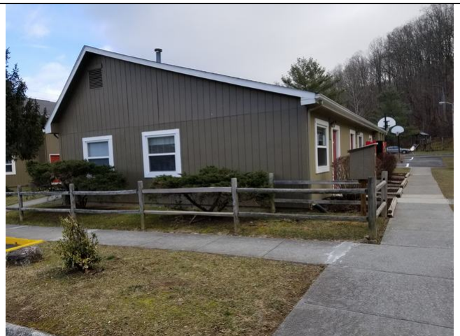
SUBJECT WALKWAY AND LEASING OFFICE
