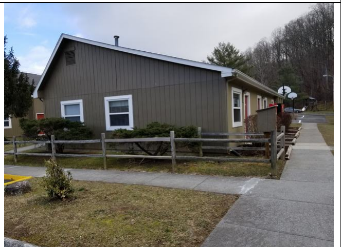
SUBJECT WALKWAY AND LEASING OFFICE
