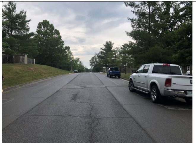
VIEW NORTH ON FAIRFAX STREET
