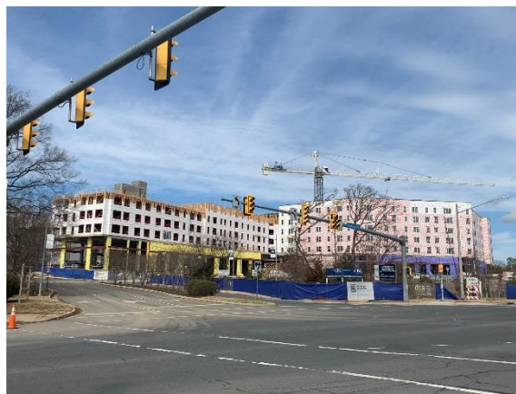
Ovation at Arrowbrook Construction Site
