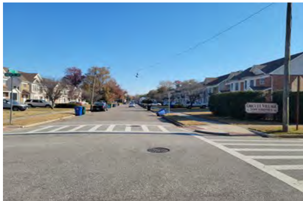
Looking East From Entrance
