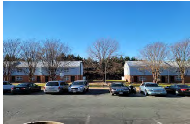
Looking West From Entrance
