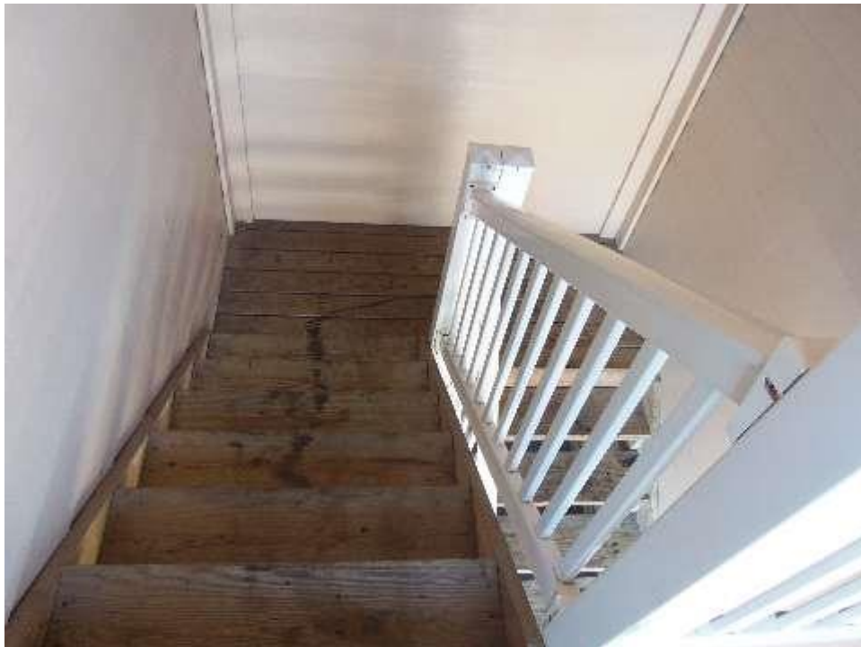
View of Typical Stairway
