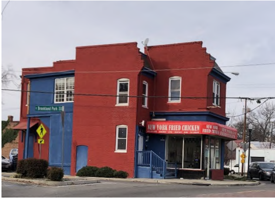
Building on the subject's side of Six Points intersection
