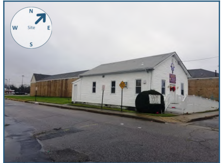
Northeast view from site
