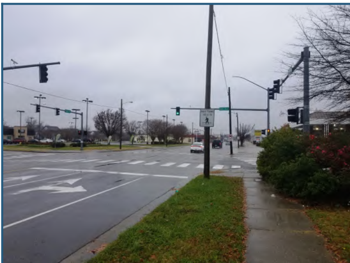
Streetscape: West view of High Street
