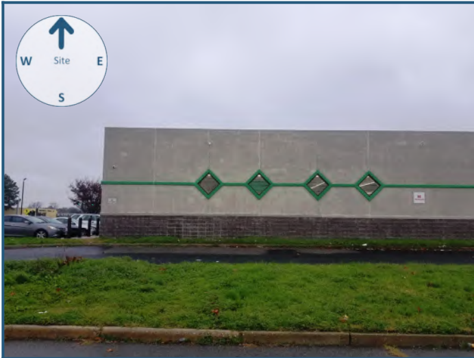
North view from site
