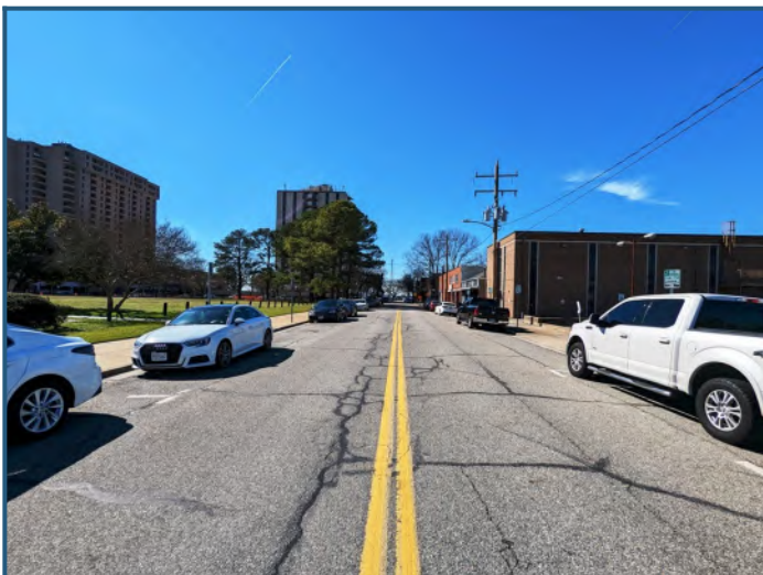
Streetscape: West view of 28th Street
