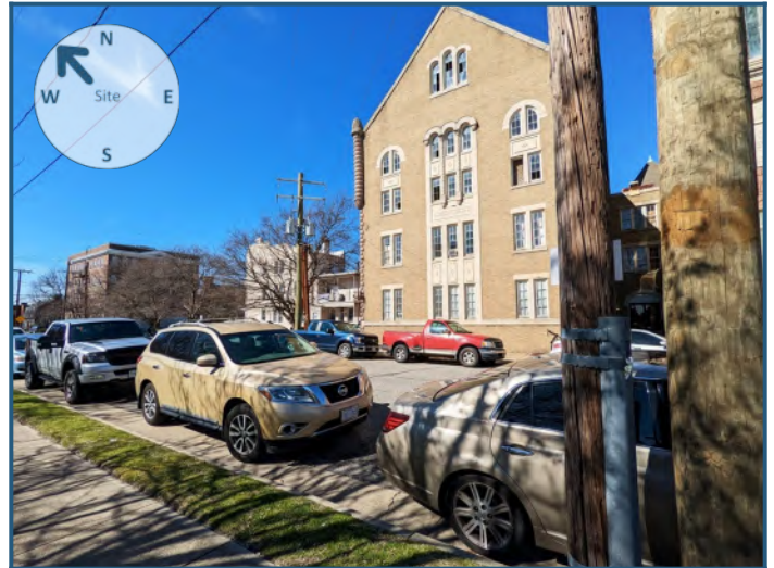
Northwest view from site
