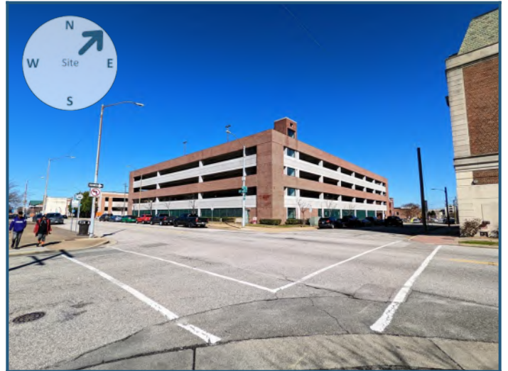
Northeast view from site
