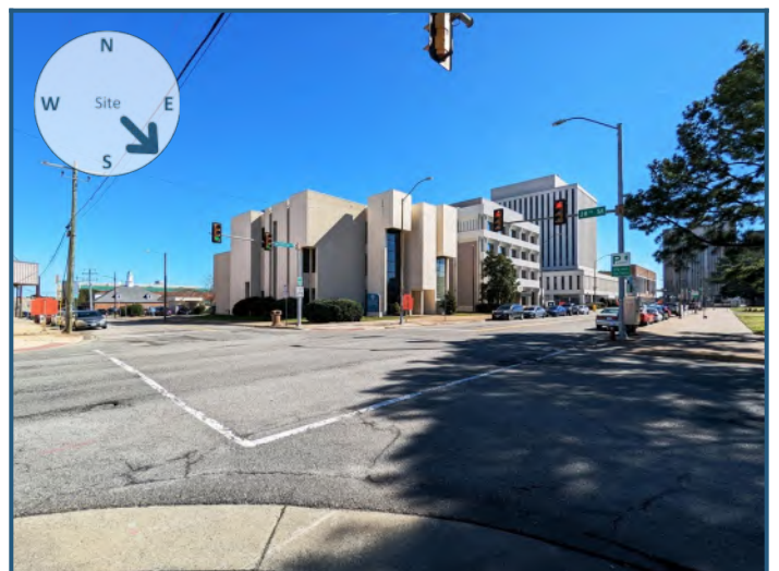
Southeast view from site
