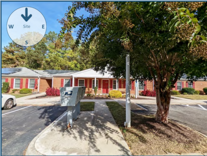
View of site from the north
