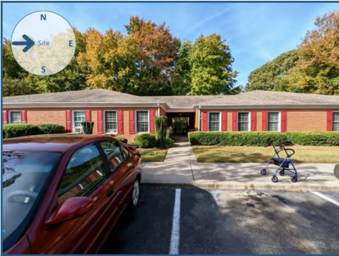
View of site from the west
