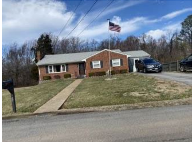
Single-family homes north of Subject site
