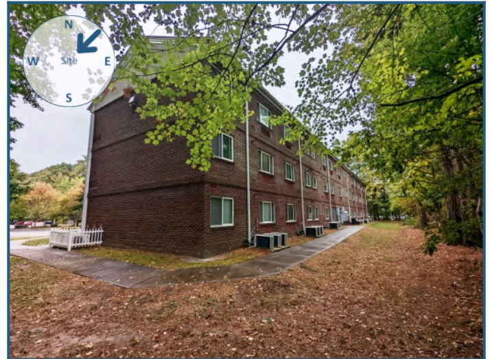
View of site from the northeast
