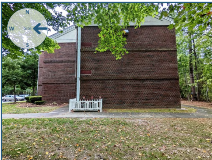
View of site from the east
