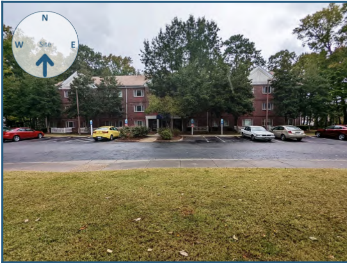
View of site from the south
