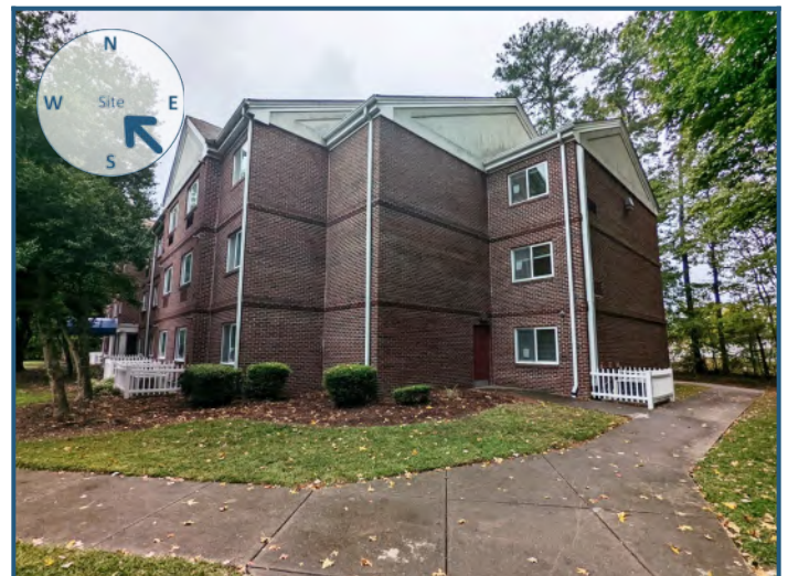
View of site from the southeast
