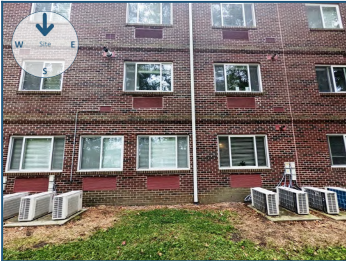
View of site from the north
