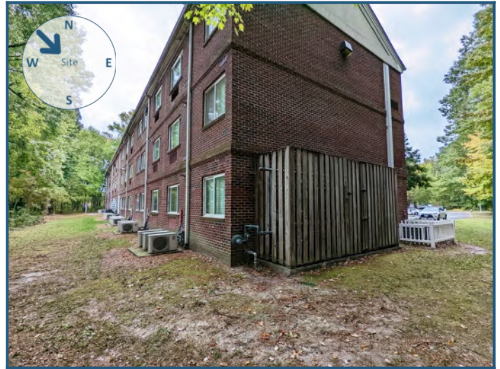
View of site from the northwest
